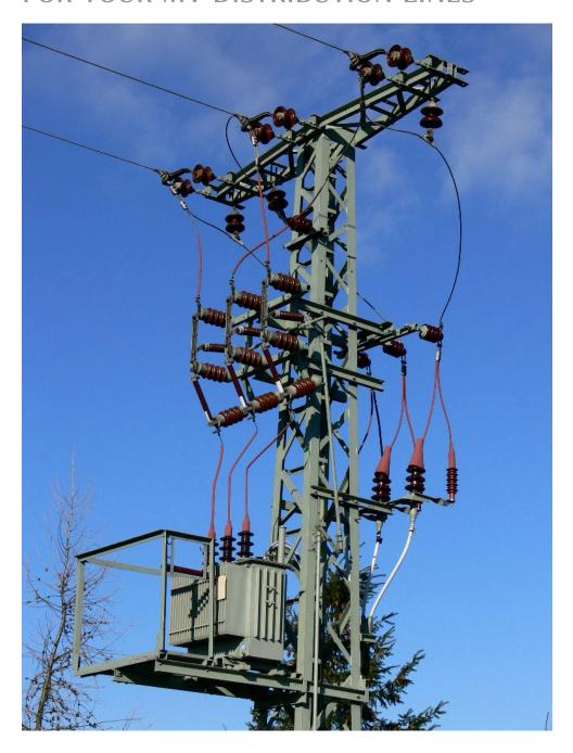
Current-limiting HV fuses are commonly used to protect branch lines in MV distribution systems in the event of short-circuit faults. Their application is specifically useful to protect overhead lines in areas of frequent thunderstorms. By rapid disconnection of a faulted branches and spur lines, they ensure optimum availability of power in neighbouring systems connected to the same feeder line.
